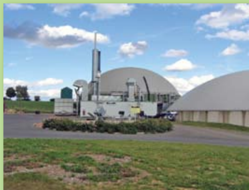
Energy production facility in the village of Jühnde, Germany.
