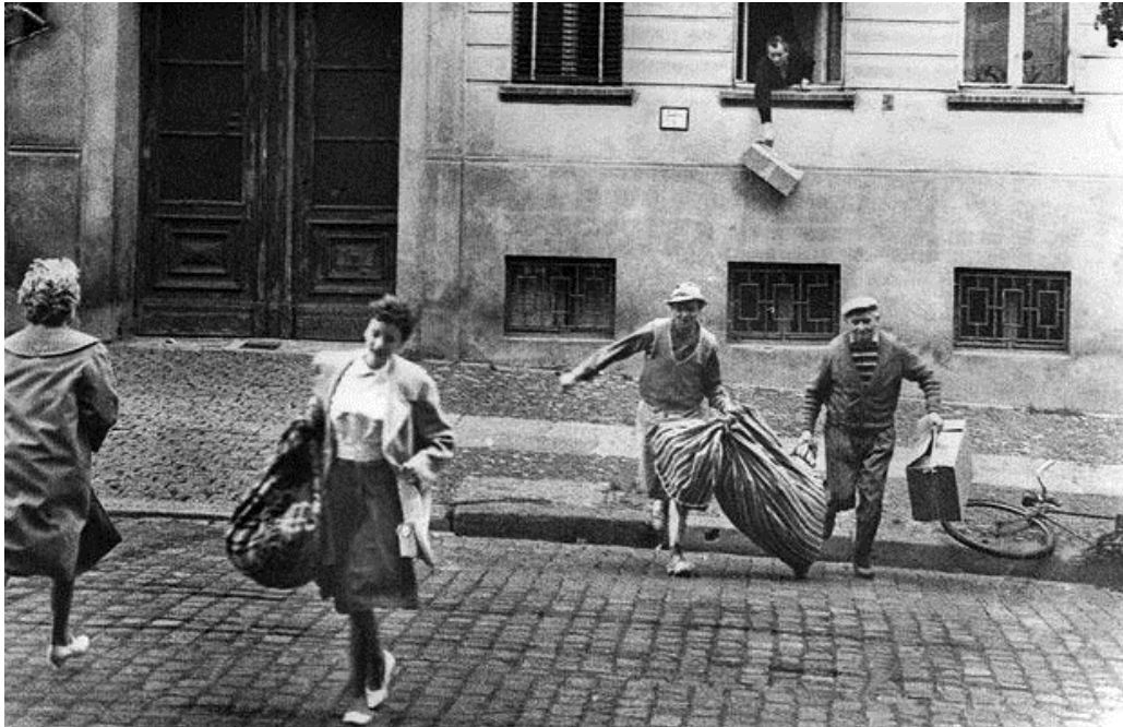
So many people jumped out of the windows on the first day of the Wall that the GDR bricked up all the windows (see photo below). Then escapees began tunneling, so the buildings were demolished permanently.
