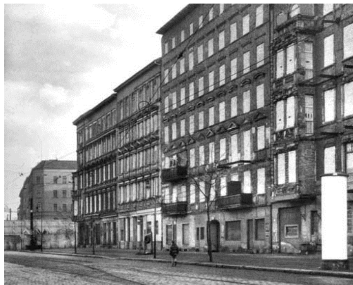
Berlin, Bernauer Strasse. The houses are situated in the East, the pedestrian is in the West. The windows were walled up to prevent people from escaping to West Berlin. (c) 2004 Heiko Burkhardt
